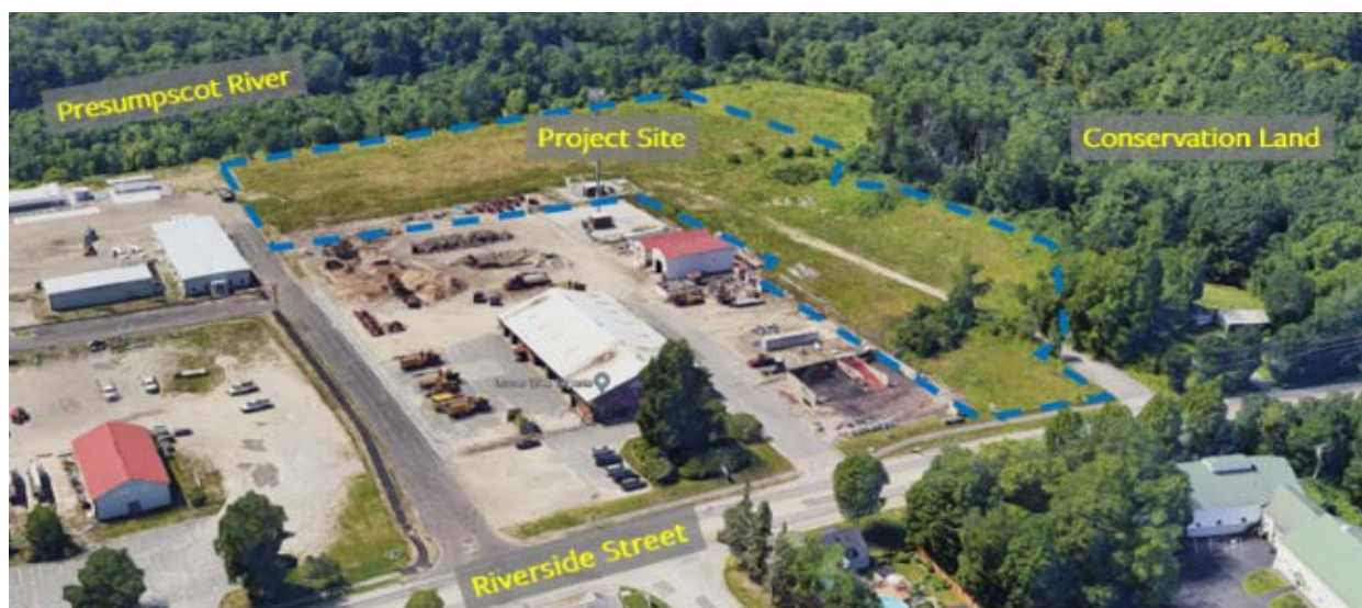
Figure 1: Project Site off of Riverside Street
