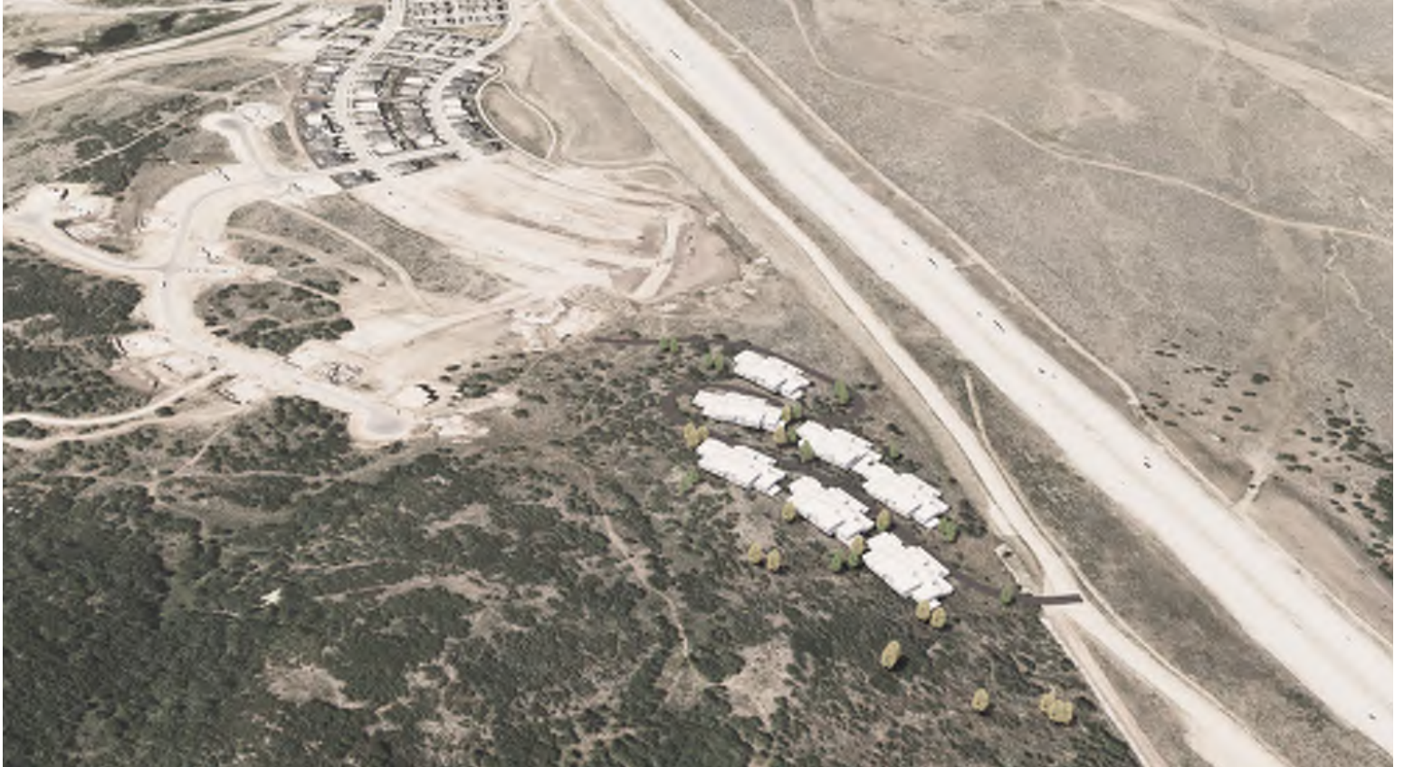
illust. 49.2 - south birdseye view looking north east towards the junction of hwy 248 & hwy 40 (Stereotomic )
