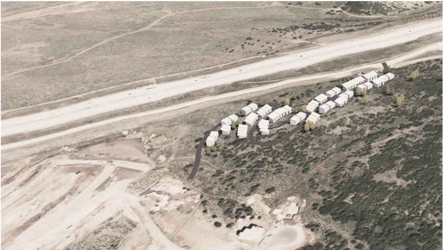
illust. 36.1 - West view of the massing as it relates to the lower hillside (Stereotomic )
