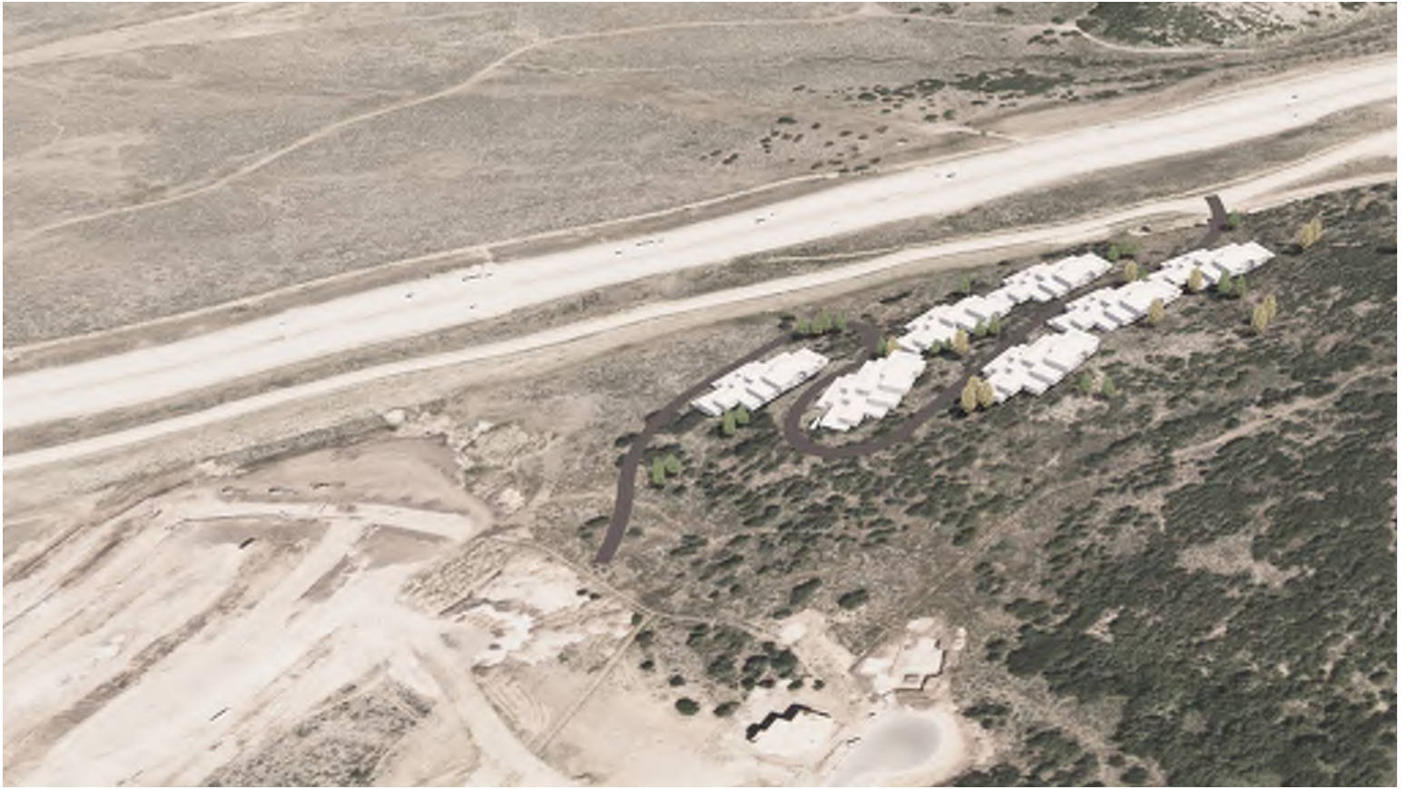
illust. 50.1 - West view of the massing as it relates to the lower hillside (Stereotomic )
