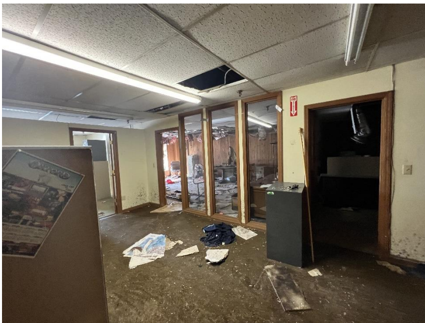
View of Second Floor non-historic trim, gypsum walls, drop ceiling and black mold, camera direction southwest.
