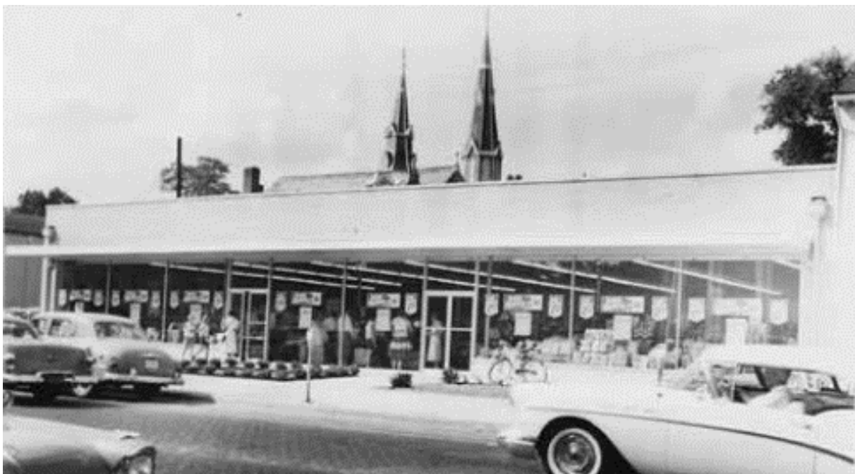
W.W. Mac Company (dime store) replaces the Girard House which was razed in 1955
