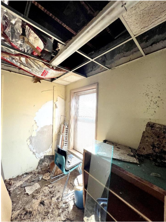
View of Second Floor vinyl replacement window, non-historic trim, gypsum walls, drop ceiling and black mold, camera direction southeast.
