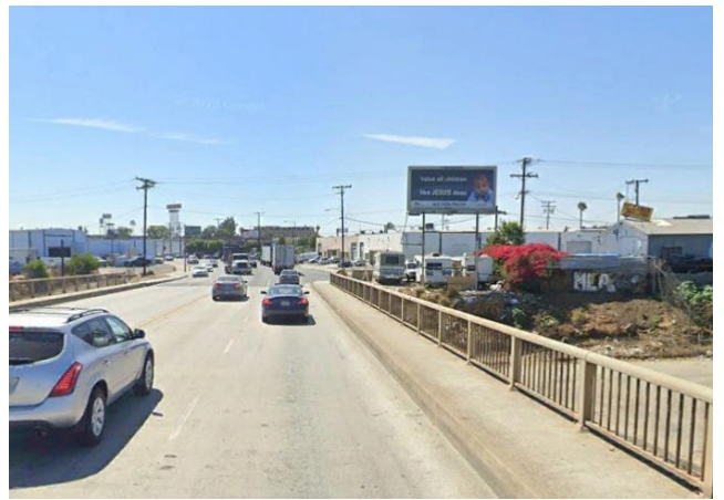
Existing East Face
