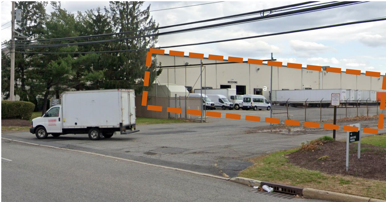
Figure 3A: Typical Warehouse in Secaucus – 250,000 Square Feet and 25 Loading Docks
