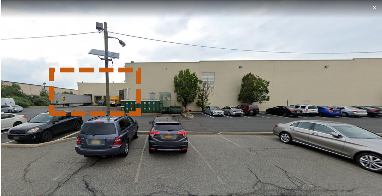
Figure 3A: Typical Warehouse in Secaucus – 125,000 Square Feet and 6 Loading Docks
