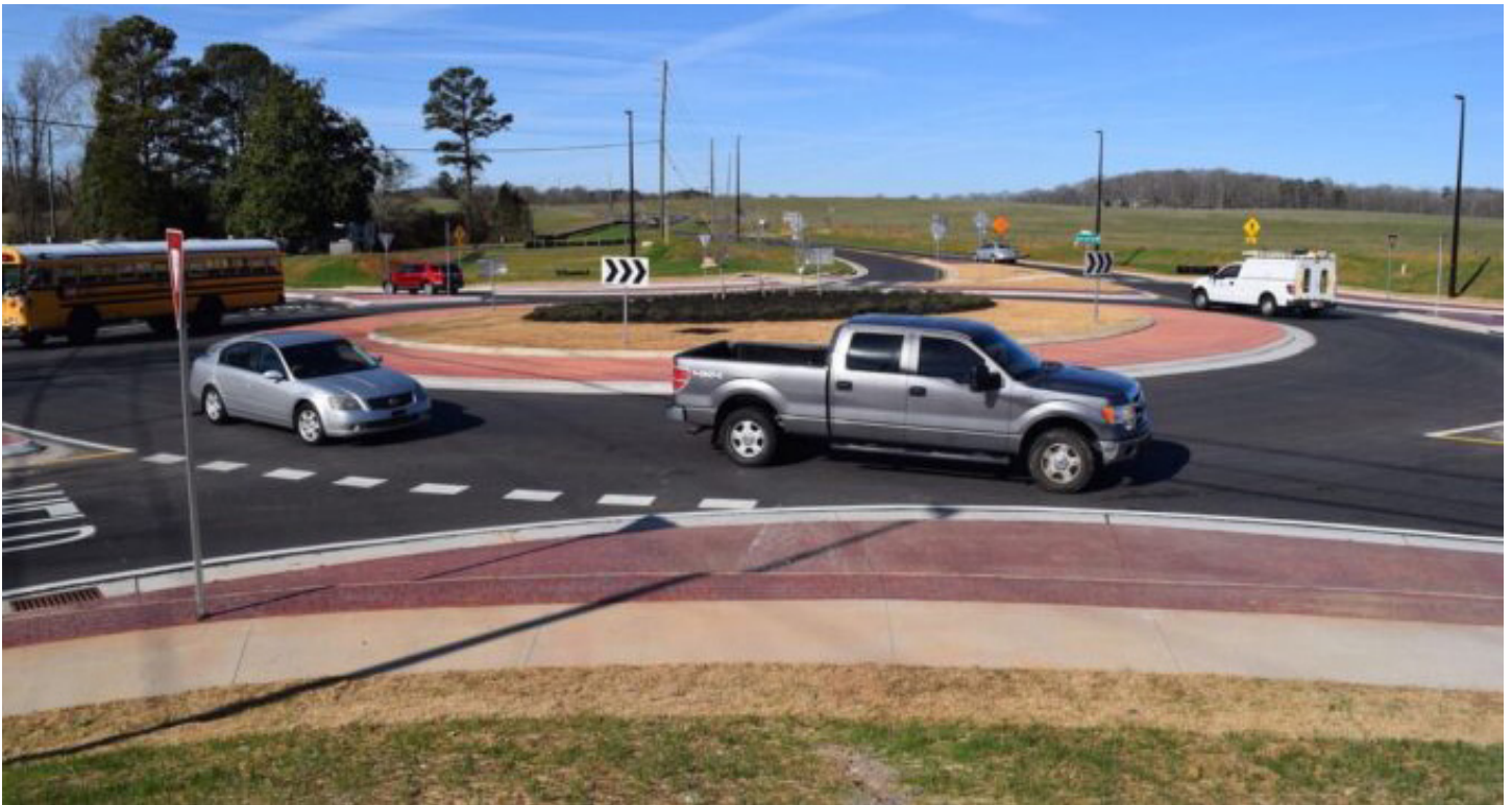
Henry County's recent roundabout investments through SPLOST Image Source: mhnews.com
