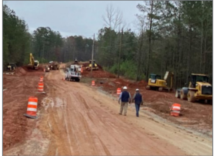
SPLOST roadway project under construction
