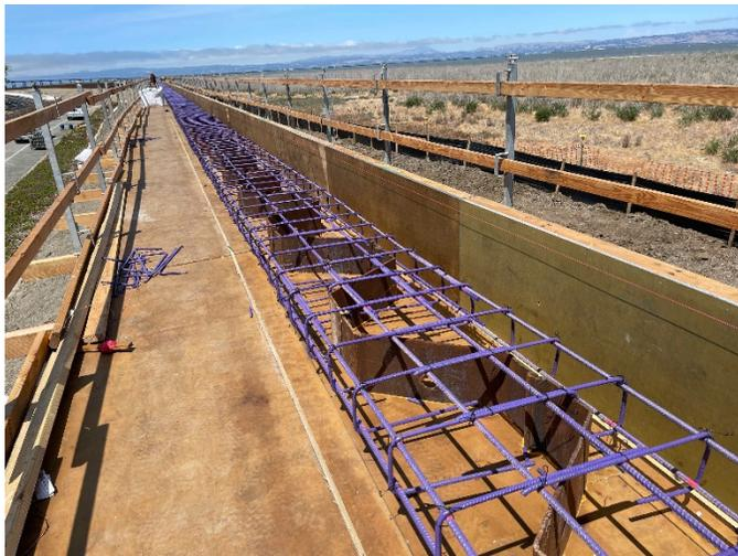
Sheet pile concrete cap reinforcement along Floodwall 12 (adjacent to Beach Park Blvd)
