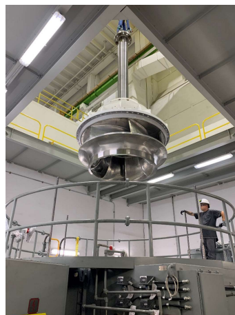
Waddell Unit 1 Overhaul
