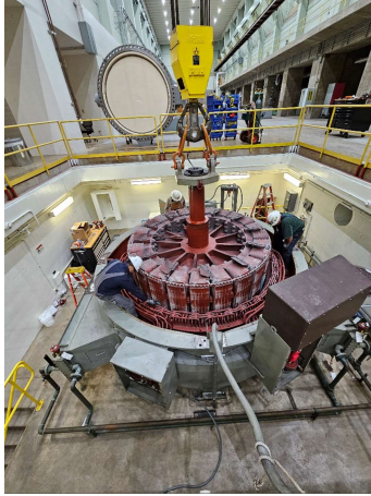
Hassayampa Unit 4 Overhaul
